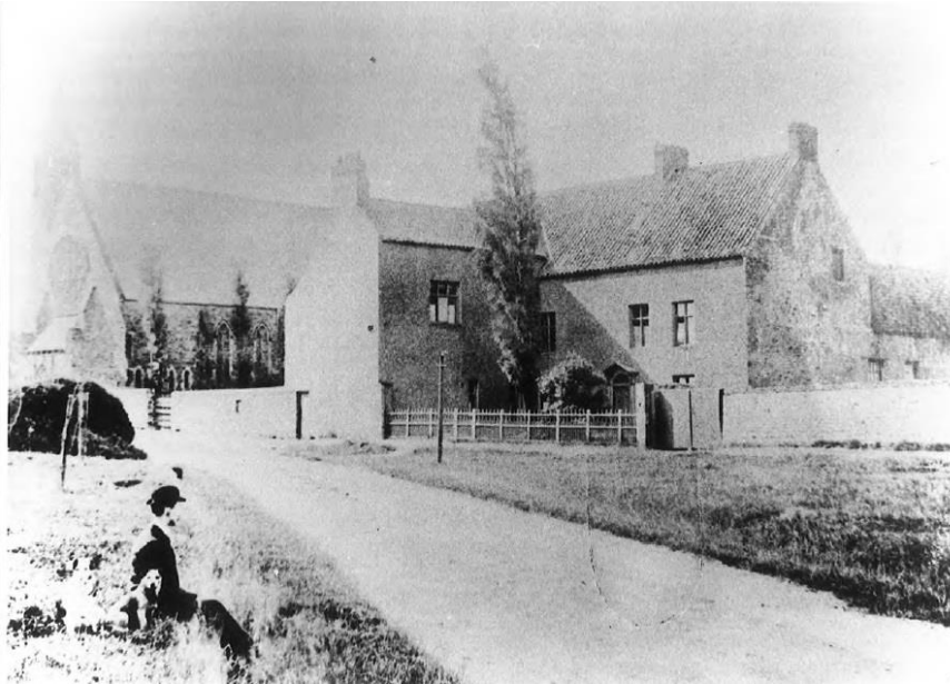
Figure 1. The Tudhoe Academy building, with St. Charles's church in the background.
